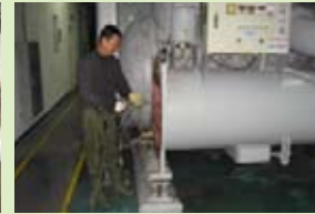
Cleaning the copper coil
